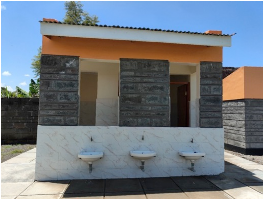
Toilets and a urinal pit
