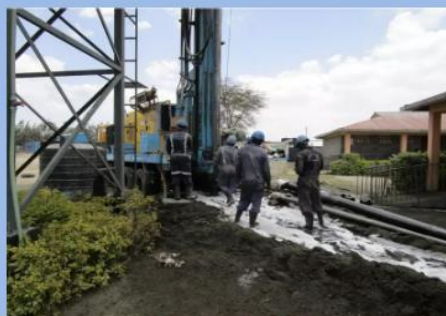
The start of well drilling
