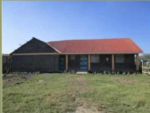
Computer lab on the left and a tailoring workshop on the right
