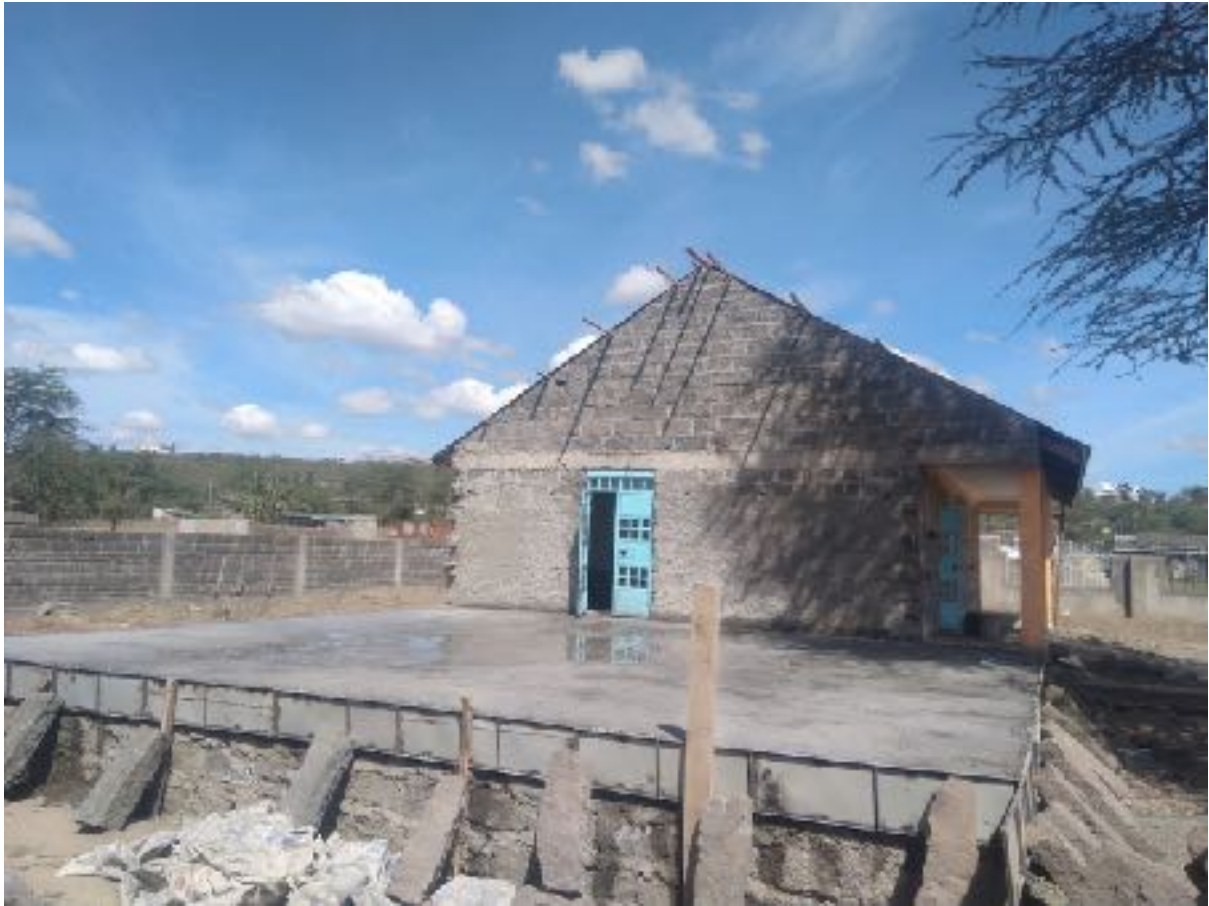
Floor slab for an IT classroom
