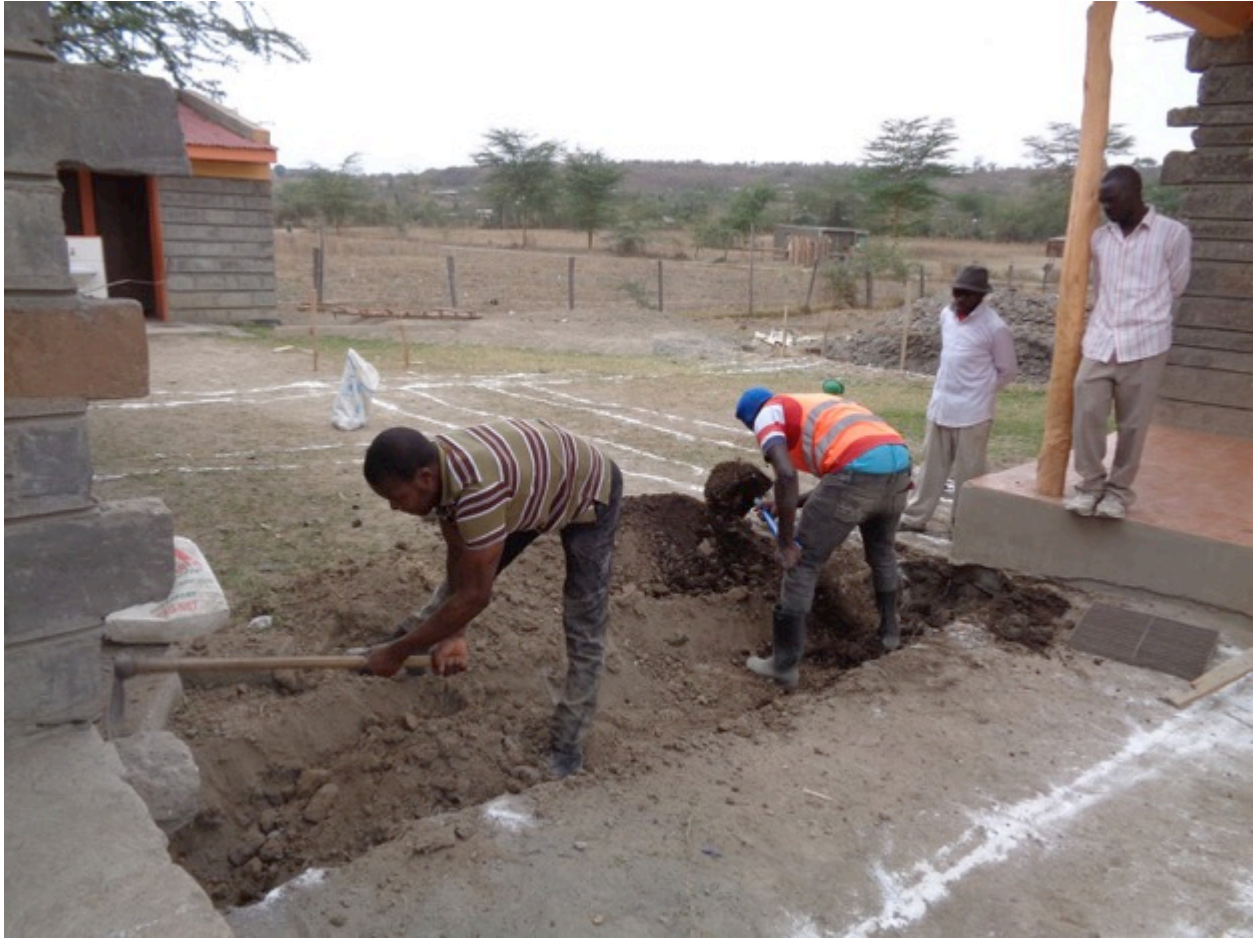
Foundation digging of the classroom on 12 th , March
