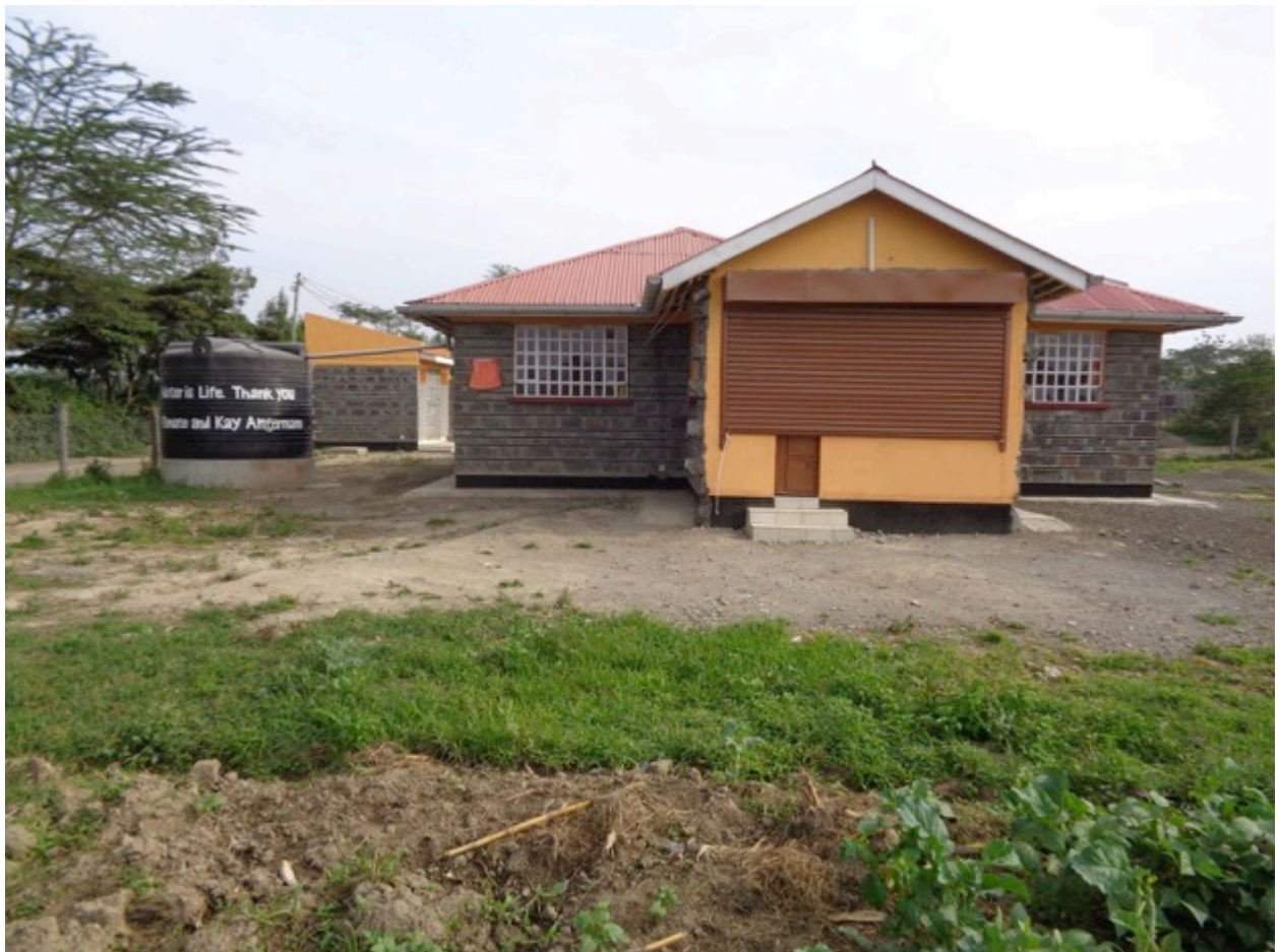
A completed modern kitchen
