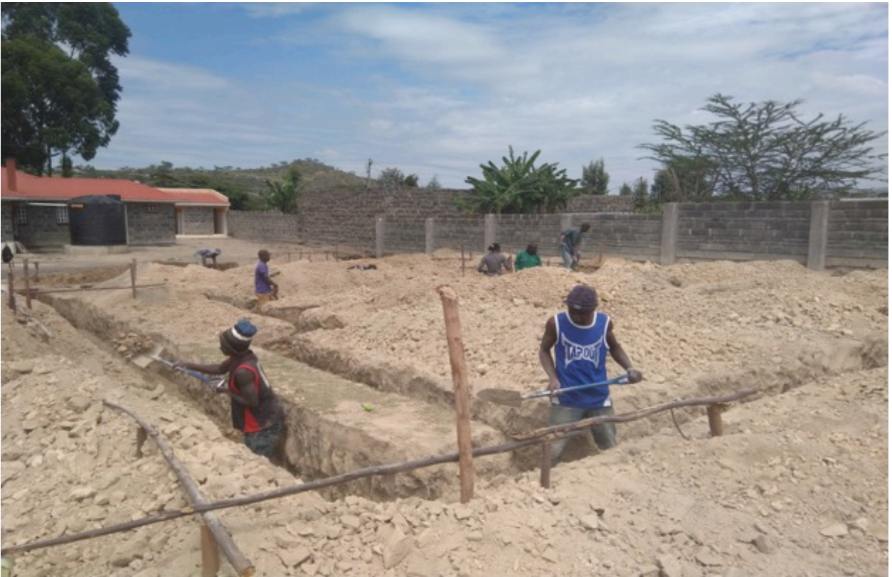
Construction in progress
