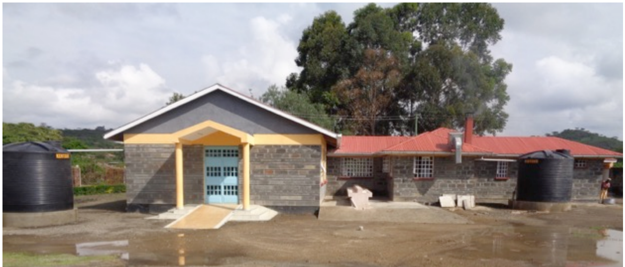
The complete dining hall, kitchen and water tanks for rain harvesting
