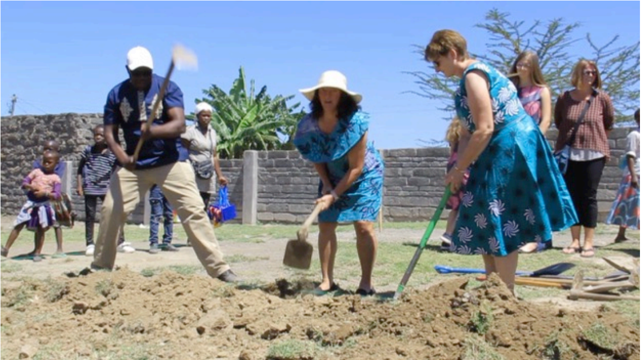
Ground breaking of Kindergarten construction
