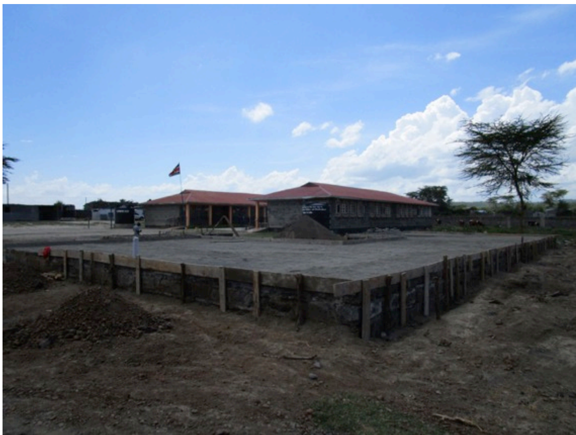
Administration, Library and Clinic block under construction – January 2020
