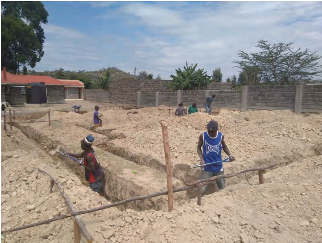
Construction in progress
