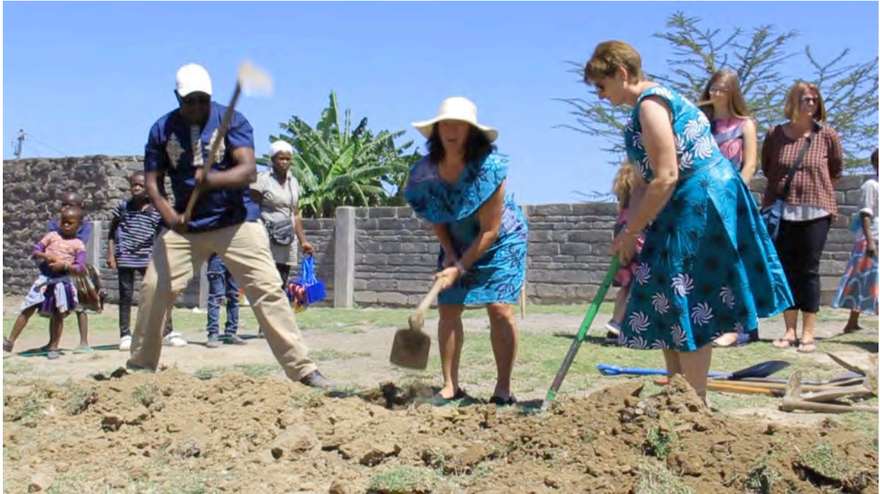
Ground-breaking of Kindergarten construction
