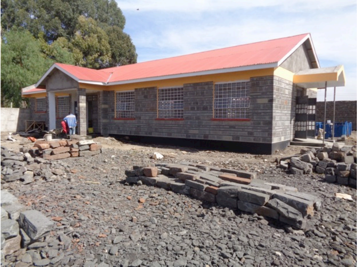
Work in progress at our dining hall
