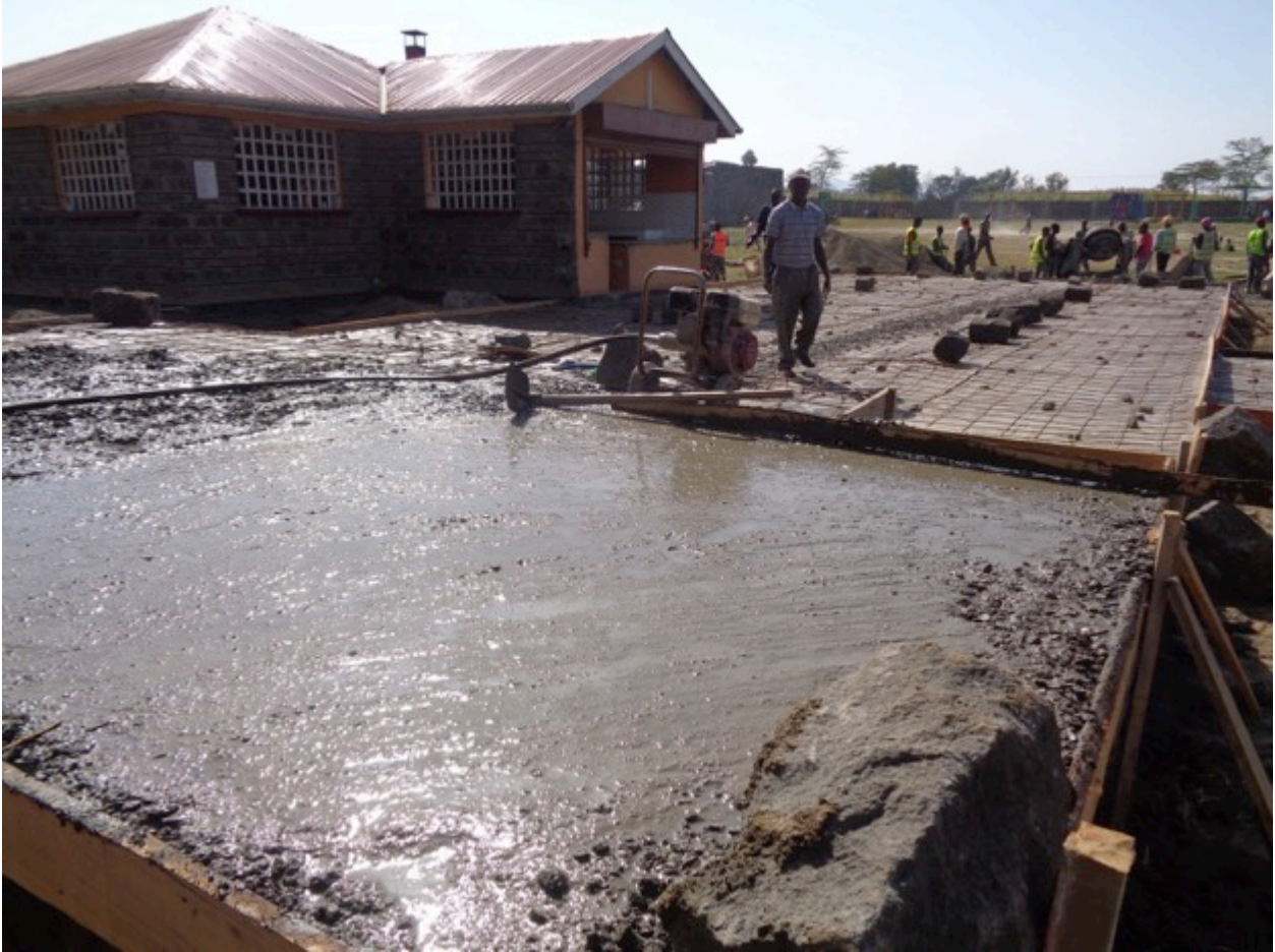
Concreting the hall floor
