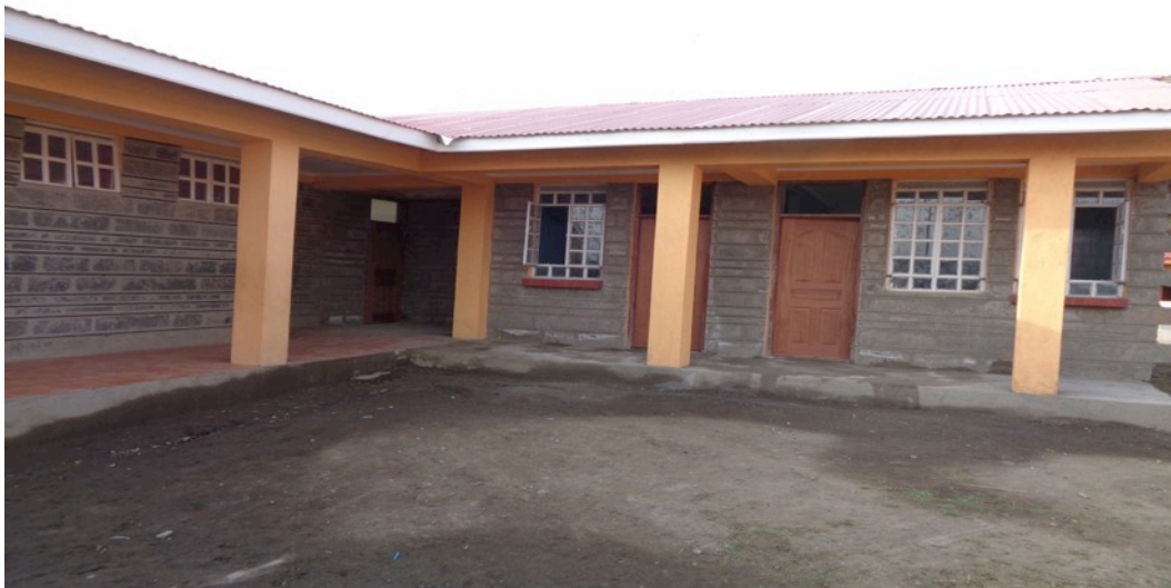
Classroom and offices construction almost ready for use
